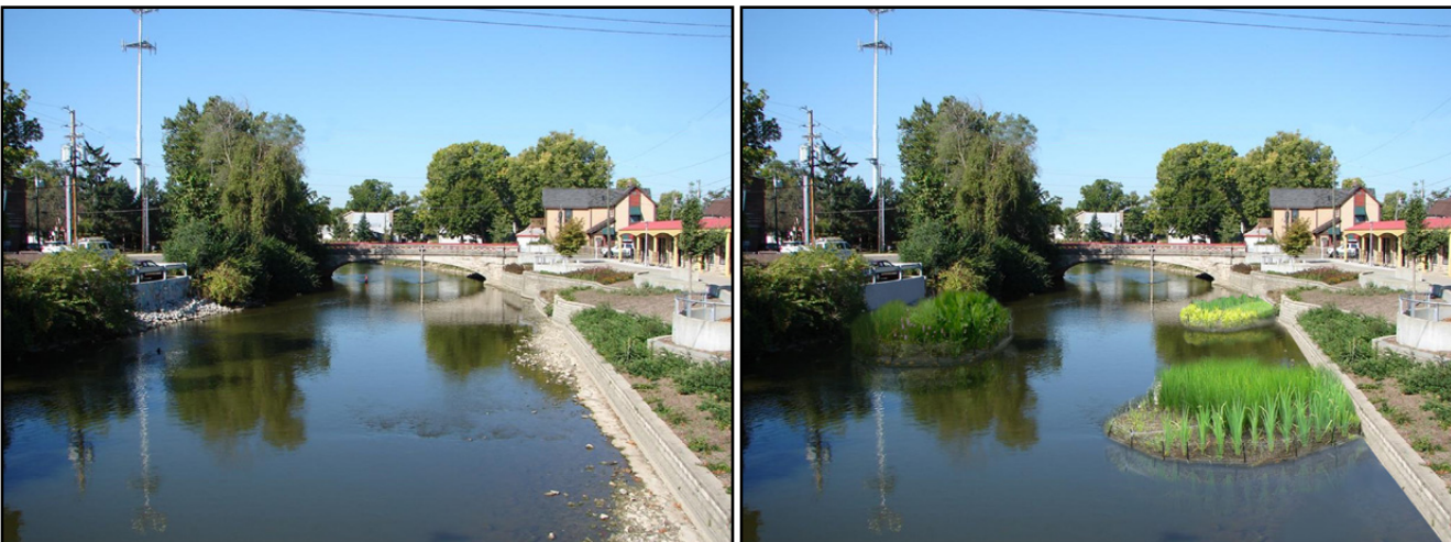
Image 6. Before and after comparison of canal with installation of floating islands
